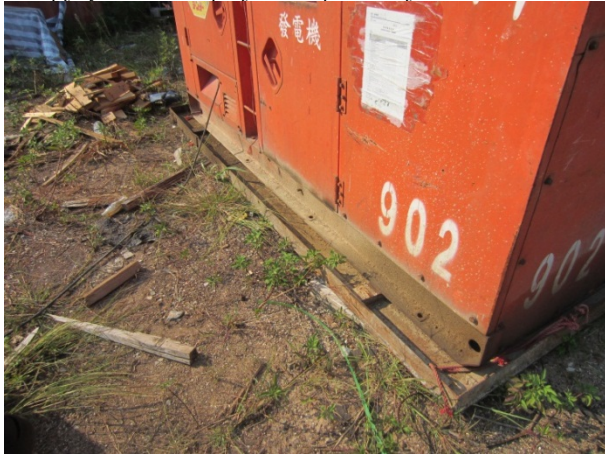
Photo 3 - A dip tray was provided for the generator that potentially has oil leakage.
