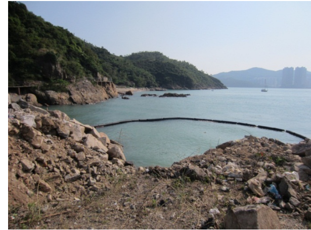
Photo 2 - A silt curtain was employed around the seawall area.
